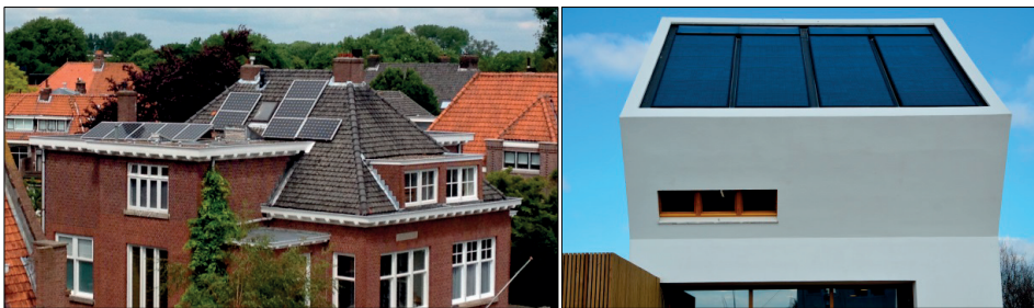
Figure 1. Free standing and roof mounted Building Added PV in Rotterdam, the Netherlands, 2013 (left) vs Building Integrated PV in Heerlen, the Netherlands, 2013 (right).
