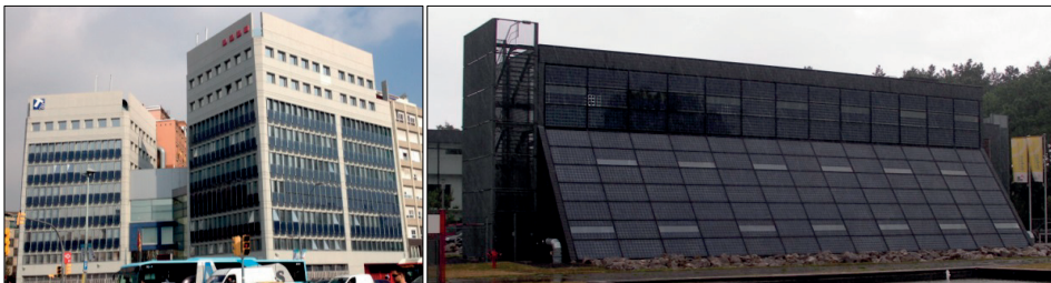
Figure 2. Two examples of BIPV on office buildings, contributing to the environmental consciousness impression of the occupants (left: office building in Barcelona, Spain, 2014, right: office building in Westerlo, Belgium, 2011).
