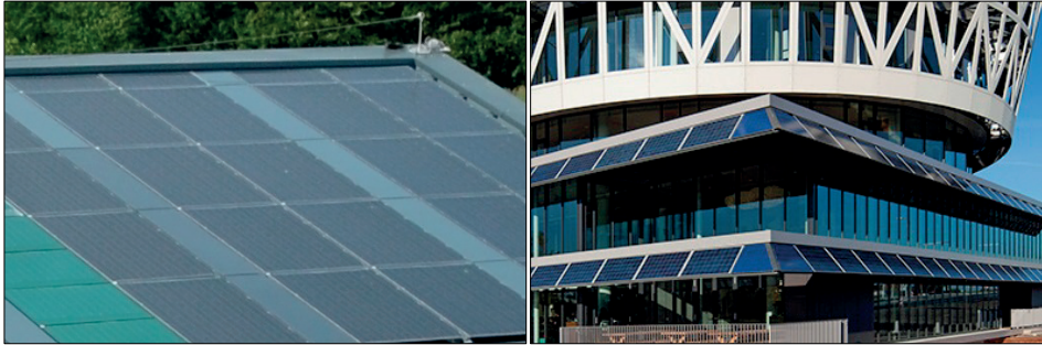
Figure 25. Two examples of BIPV dummies, contributing to a homogenous building skin. (left: dummies in the top row of an experimental building in Heerlen, the Netherlands, 2014, right: dummies on the corners of an office building in Roelofarendsveen, the Netherlands, 2012, reproduced with permission by Luuk Kramer).
