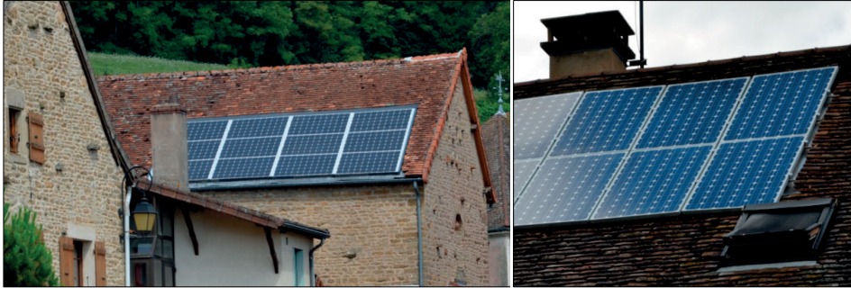
Figure 3. Two examples of BIPV systems in France (2013) in which the modules are from a technical point of view integrated in the building skin, but the aesthetic integration is lacking.
