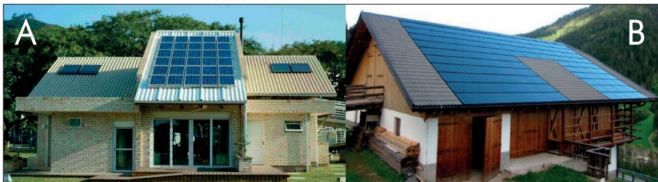
Figure 1. Photograph of rooftop BAPV realized in Florianopolis, Brazil (A) [5] and photograph of rooftop BIPV realized in Badia, Italy (B) [6].
