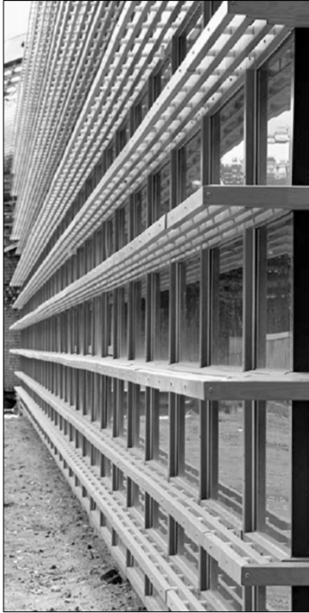
Figure 3. Picture of the realised façade retrofitting of the WNF. (vd Meijden)
