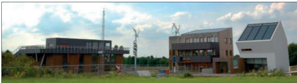
Figure 3. Picture of The District of Tomorrow (TDoT) with three realized innovative building objects, with at the right field test 1.
