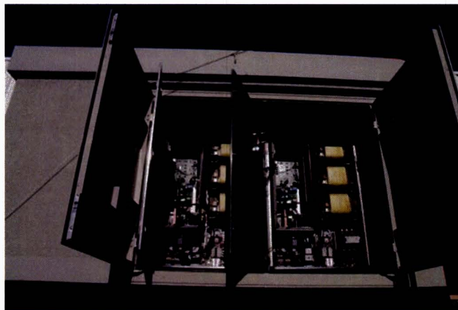
Figure 2.3 Photo of the two inverters of the BESS at Etten Leur, seen from the side-door.
