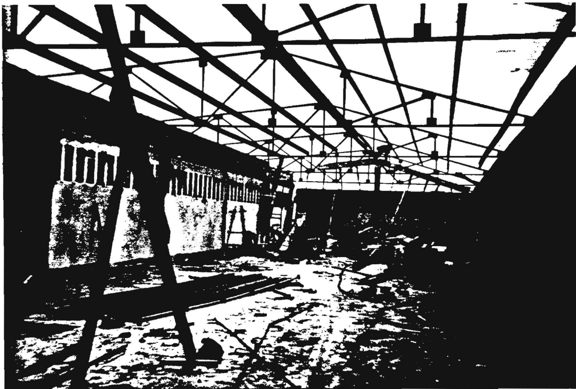
Figure 9. The new building under construction.
