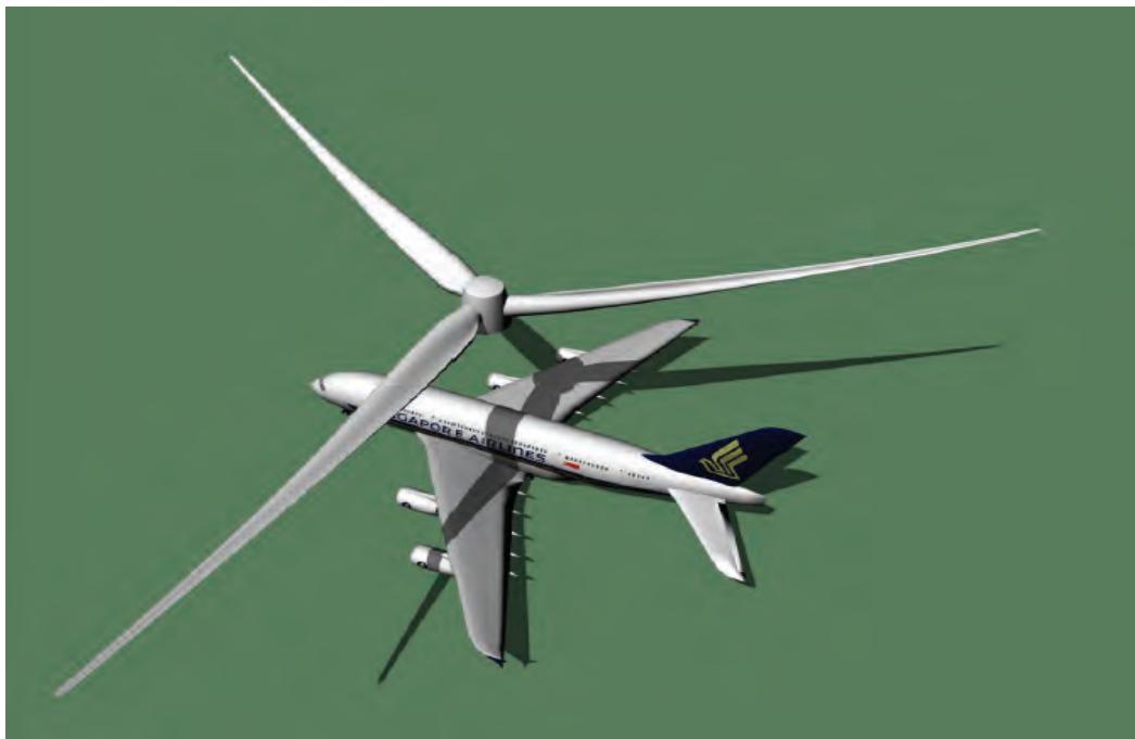
Figure 41: Gearless Siemens SWT-6.0 wind plant. Comparison of the 154 m rotor with the Airbus A 380
