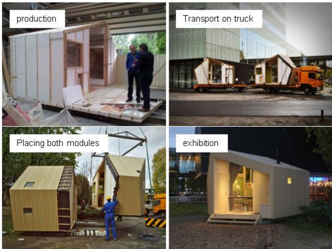
Figure 6. industrial production, transportation and placing.
