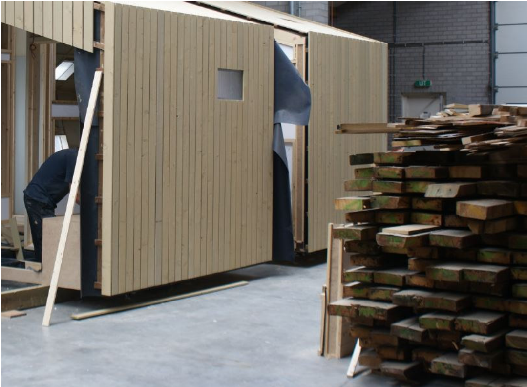
Figure 2. The Trek-In is fully build of-site, mainly made of reclaimed wood
