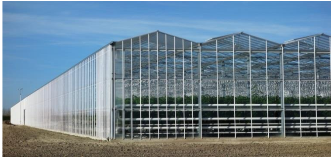
Figure 5.1 A typical Venlo-type greenhouse growing tomato crop ( www.horconex.nl )
