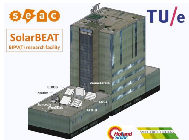
Figure 2: Sketch-up model of the complete research facility shows the various project names. The model is also used for shading analysis.
