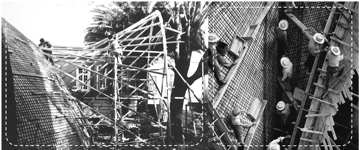
Figure 4: formwork construction by Felix Candela 2
