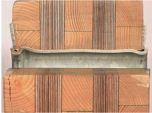
Figure 5: Three member connection with dvw glued to the timbers separately at the shear planes of the expanded tube.
