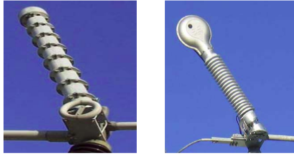
Figure 2.11. (Left) multiple vacuum interrupters and (right) a single gap SF 6 interrupter per phase (copied from [45]).
