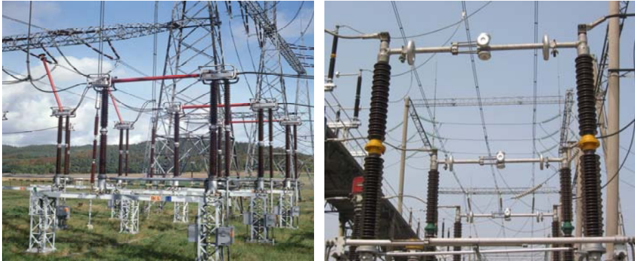
Figure 1.1. (left) A three-phase vertical-break DS mounted horizontally in a closed position (Courtesy of HAPAM B.V.); (right) centre-break DS in a closed position (Courtesy of Siemens).
