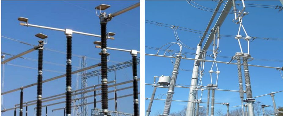
Figure 1.2. (left) Double-break DS in an open position; (right) pantograph DS in a closed position (Courtesy of HAPAM B.V).
