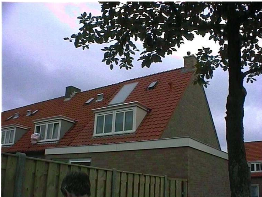
Figure 9 Renovated roof with PV panel
