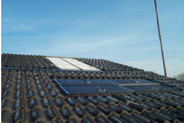
Figure 4: full scale experiment on solar panels integrated in tiled roofs.
