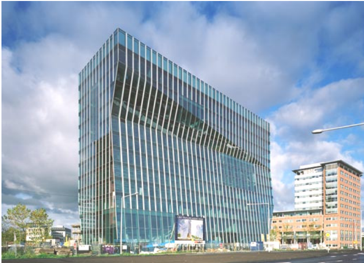
Figure 1.4: Glass panes as tertiary structural elements in a façade structure (assurance company Atradius, Amsterdam, The Netherlands)
