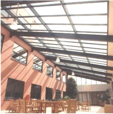
Figure 1.3: Glass panes as tertiary structural elements in a roof structure (King Fischer BCC, Amsterdam, The Netherlands)
