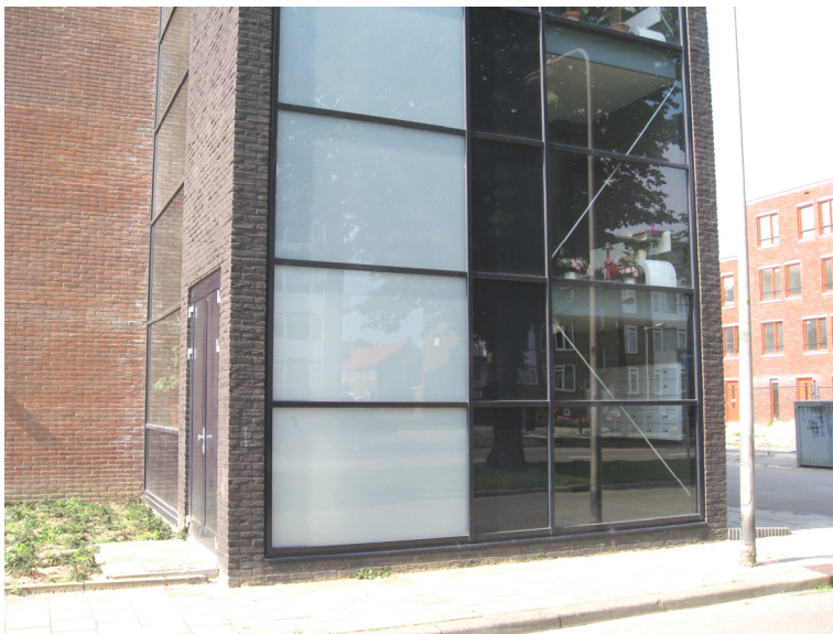
Figure 1.9: Steel braces behind glass façade of a residential building, Arnhem, The Netherlands
