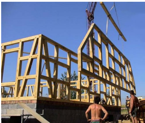
Figure 1.36: Assembly of a timber-framed wall
