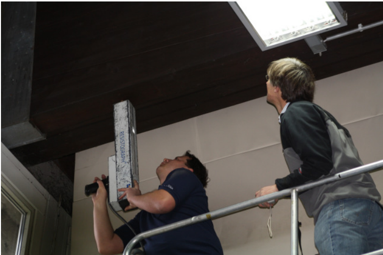
Figure 3.28: Inspection of the binder support points using the resistograph
