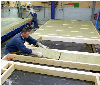
Figure 1.40: Manufacturing of a prefabricated wall in timber frame design
