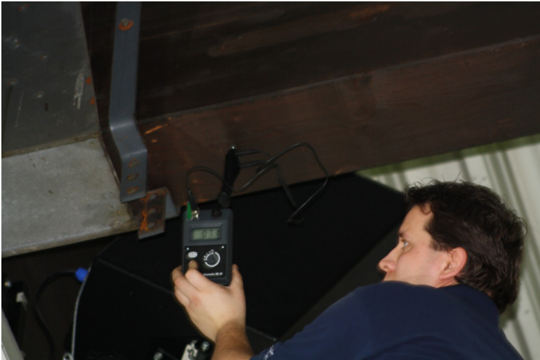
Figure 3.30: Electrical wood moisture test
