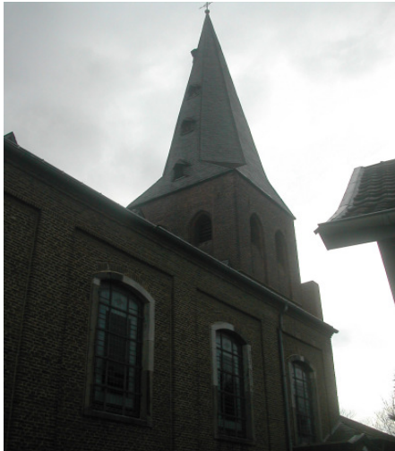
Figure 3.2: Photo – Church tower with aisle
