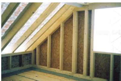
Figure 1.17: Typical use of chipboards as cladding for timber frame constructions
