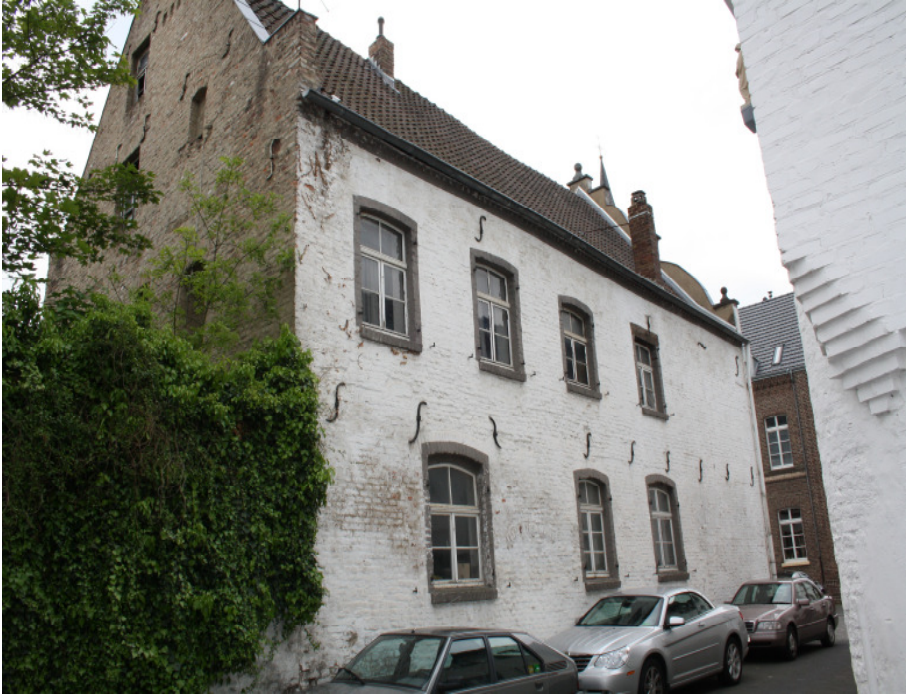
Figure 3.10: Photo – Side view of the building
