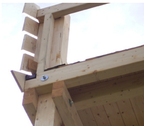
Figure 1.55: Mechanical connection resource: Special dowel design
