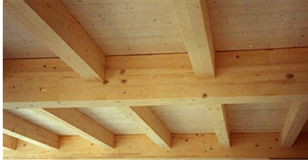
Figure 1.33: Wooden-beam ceiling in visible implementation
