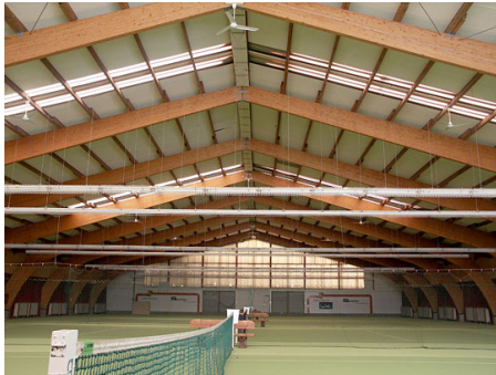
Figure 1.48: Inside view of a lunging hall in Unken (Austria) with supported three-dimensional wood construction
