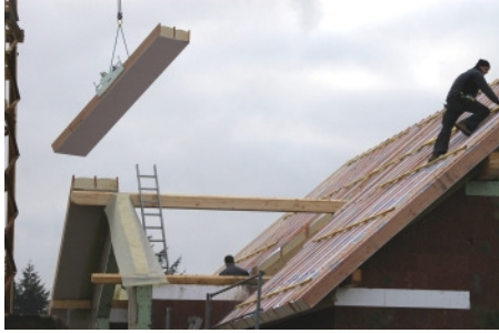
Figure 1.35: Assembly of a pre-manufactured heat-insulated roof element
