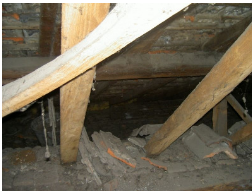
Figure 1.65: Wooden wind brace on bottom side of the rafter
