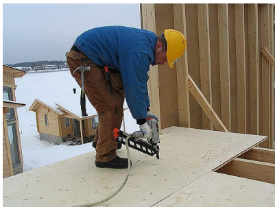
Figure 1.15: Typical use of spruce plywood sheets as formwork for a wooden-beam ceiling
