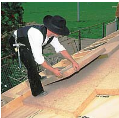
Figure 1.19: Typical use of wood fiber boards as insulation material for rafter insulation = insulating wood fiber board
