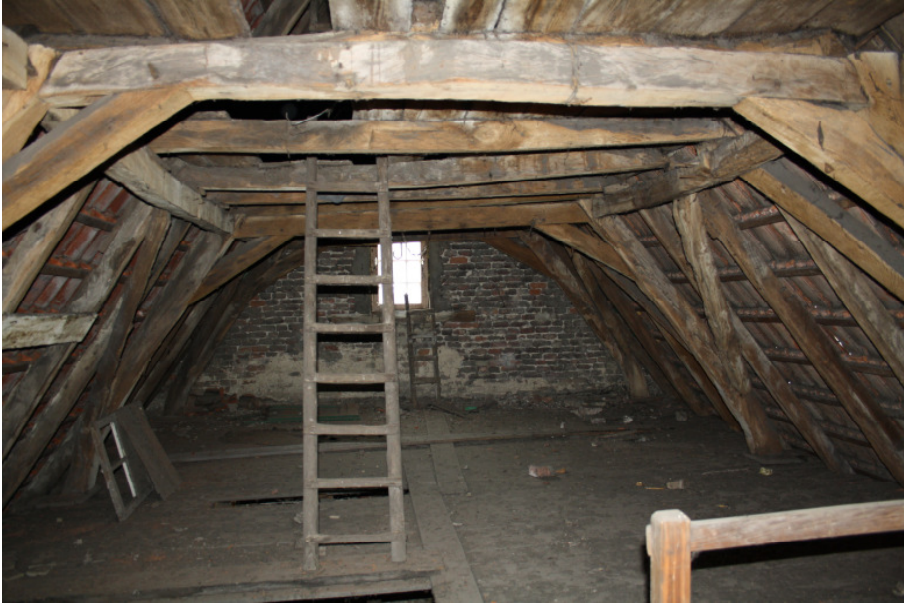
Figure 3.15: Photo – Level 2 of the roof construction
