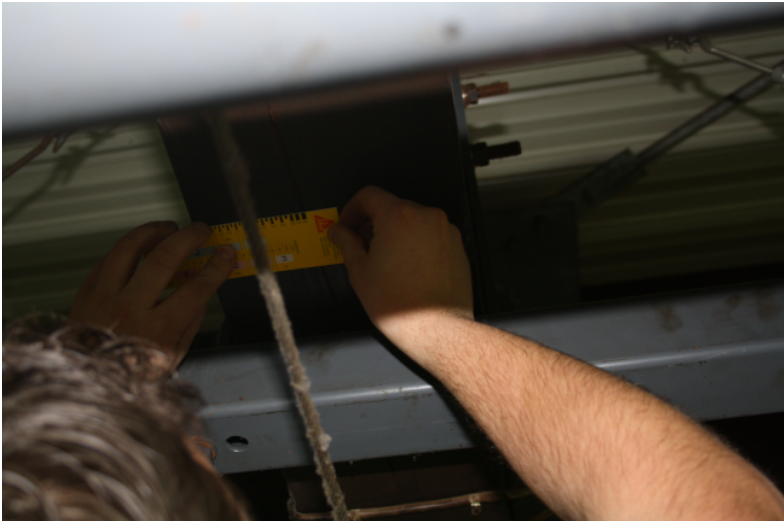
Figure 3.29: Inspection of a crack using a crack gauge
