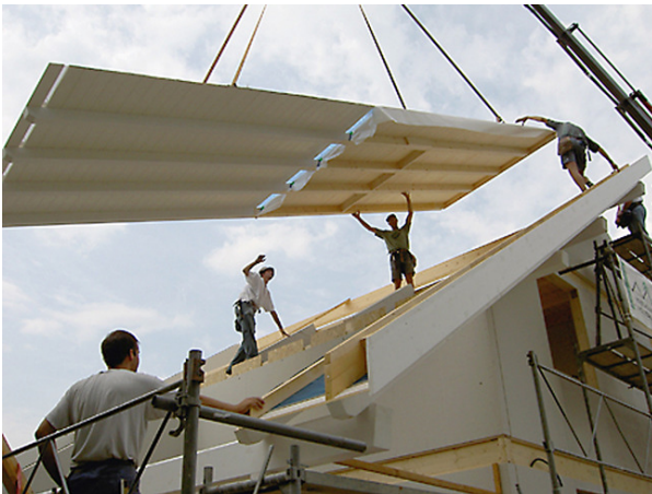
Figure 1.42: Installation of a prefabricated roof element of a prefabricated house
