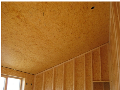
Figure 1.21: Typical use of OSB boards as windproof (= outer) sealing level of a passive house
