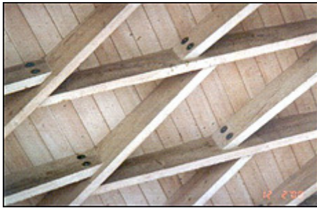
Figure 1.59: Roof panel in Zollinger construction, source [2]
