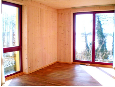
Figure 1.43: Inside view of a board stacking ceiling and wooden plank wall
