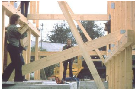
Figure 1.54: Different engineered connections with sheet metal parts
