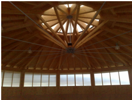
Figure 1.49: Bottom view of the supporting structure (see figure 1.48) with an engineered connection
