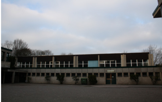
Figure 3.21: Photo – outside view
