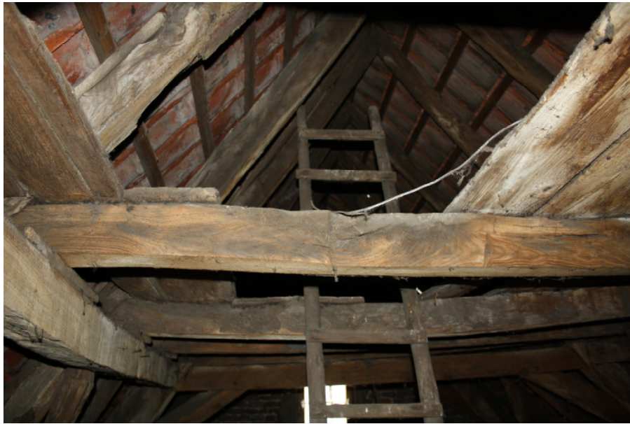
Figure 3.16: Photo – Transfer from level 2 onto level 3
