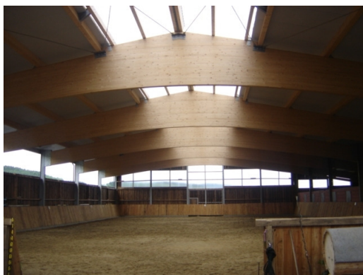
Figure 1.10: Glued laminated timber as ridged roof girder with curved underside in an indoor riding ring.
