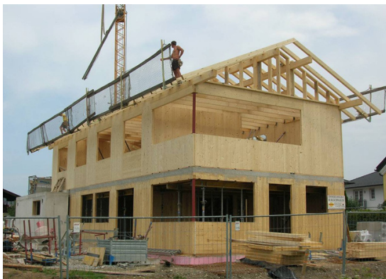
Figure 1.44: Residential house built using the board plywood construction method
