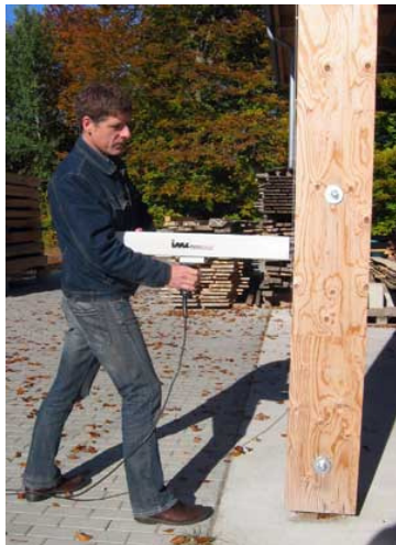
Figure 2.11: Drilling resistance measurement on a damaged supporting structure
