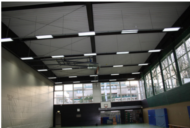
Figure 3.22: Photo – view of roof from below with roof bracing
