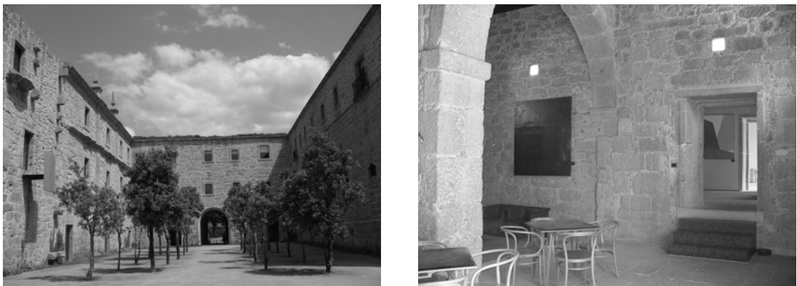
Figure 2 – Re-adaptation of a convent into a hotel, St. Maria do Bouro - Portugal, Architect Eduardo Souto de Moura e Humberto Vieira (1989 – 1997)
