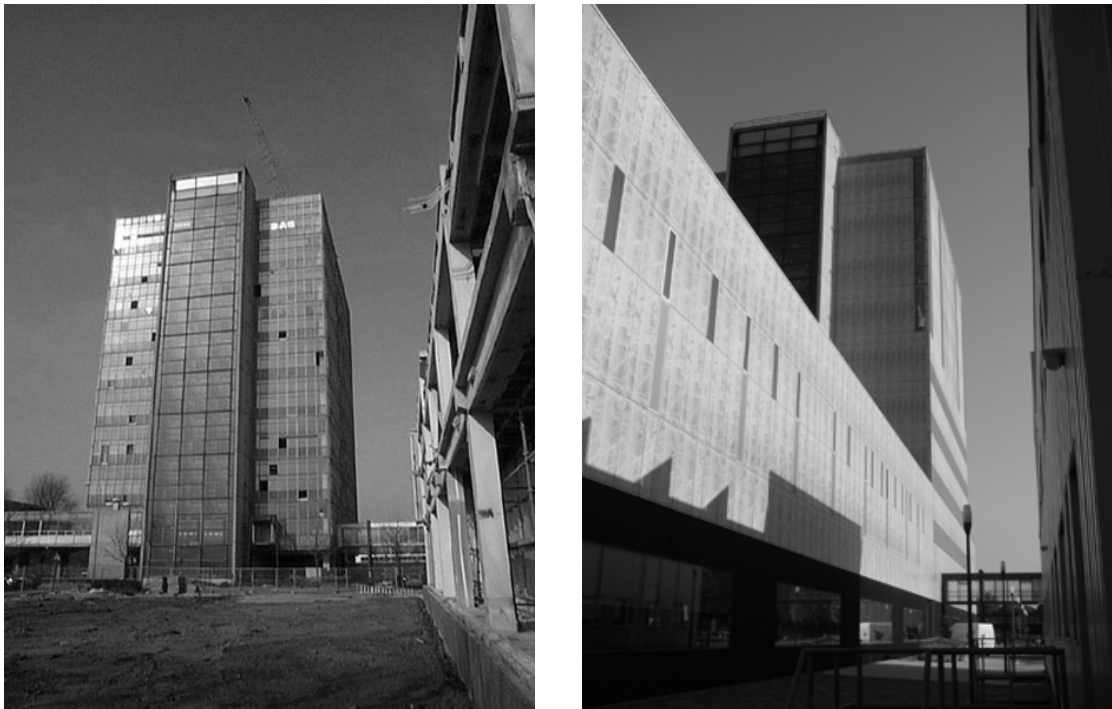
Figure 3 - Vertigo building before and after intervention (2000 – 2002) 3
