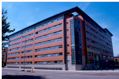
Figure 10: 9-storey modular building in Manchester
