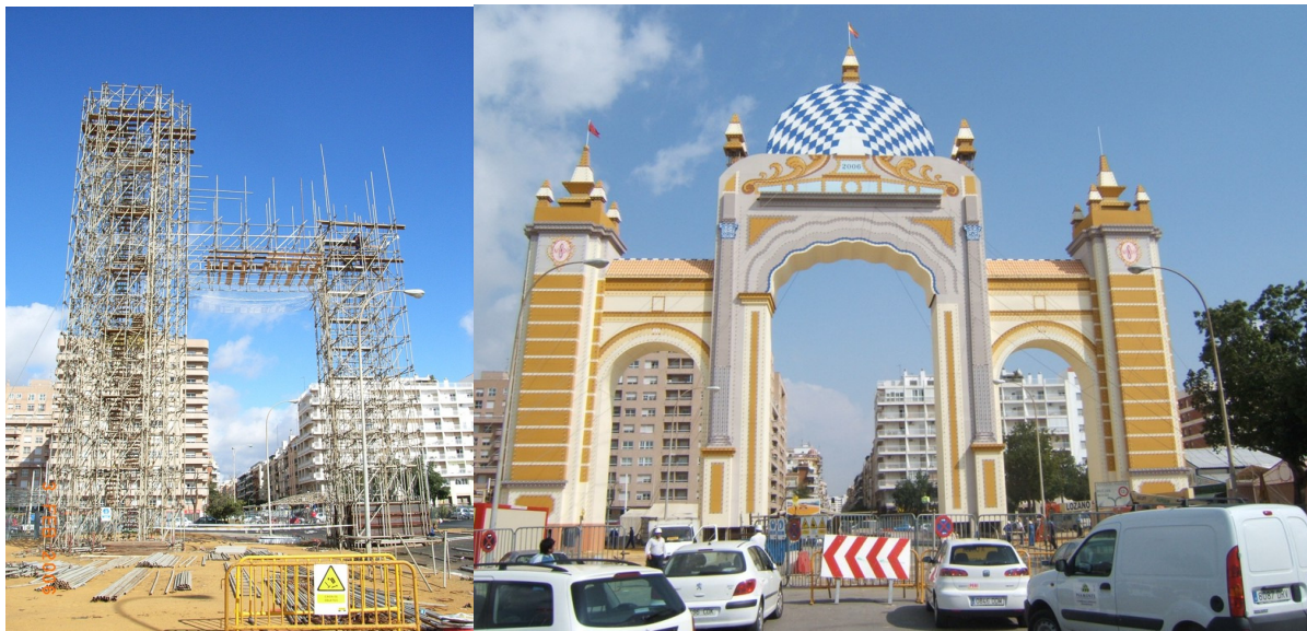
Figure 16 Building process of the 2006 gateway.
