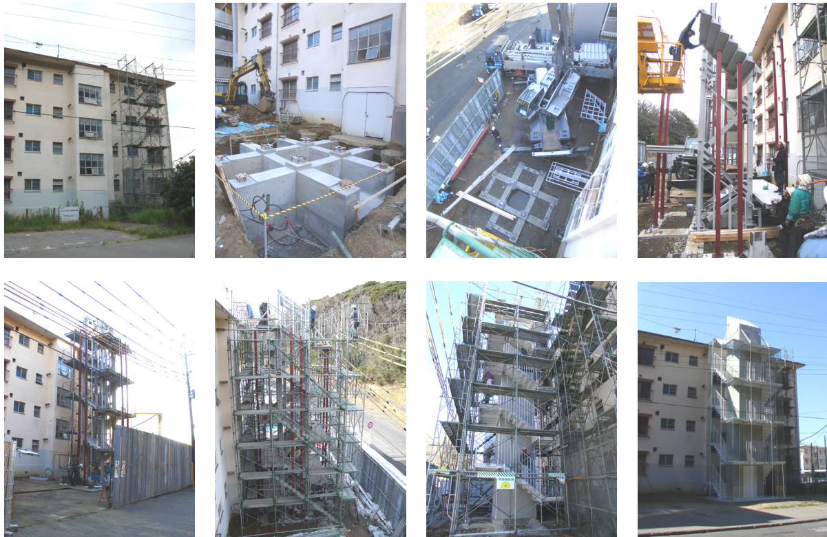
Figure 4. Process photographs of construction site
