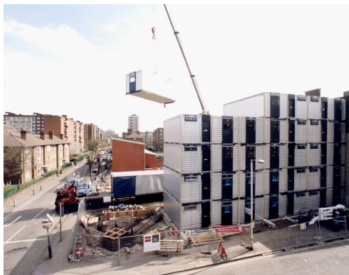
Figure 3. Murray Grove module installation
