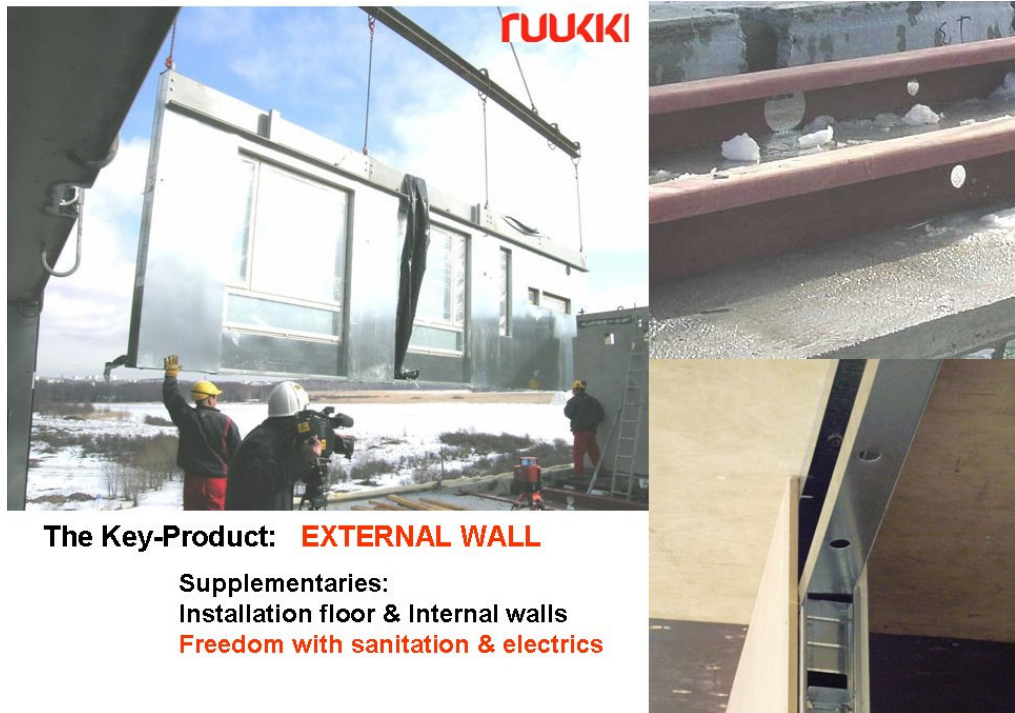
Fig.3 The pilot project allow high flexibility by advanced steel constructions
