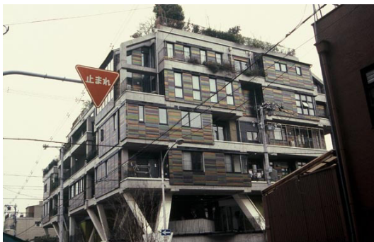
Figure 9. NEXT21 External Wall
