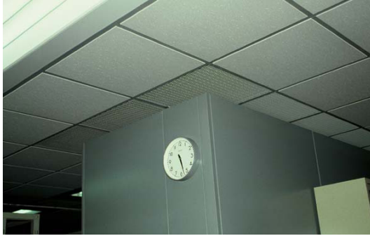
Figure 5. Ceiling panels and partitions
