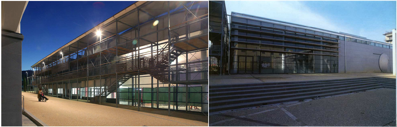
Figure 6. The east elevation: the “scaffolding” (view axis) and north elevation: vertical modules,
