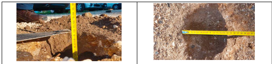
Fig. 4. Potholes dug in the parking lot annexed to the school of Engineering of Sapienza-University of Rome. a) Pothole depth; b) Pothole diameter.
