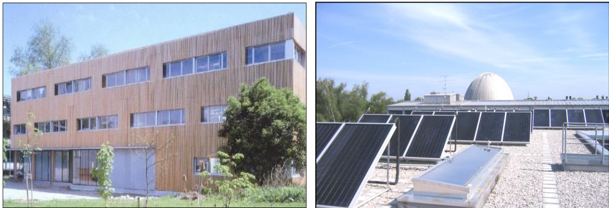
Figure 3: ZAE Bayern office building and solar thermal flat plate collectors on the rooftop
