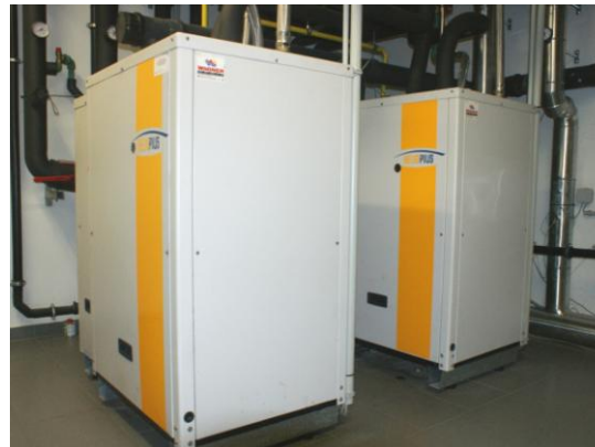
Figure 2: Photo of AHP installation
