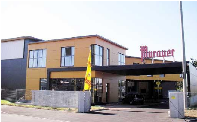
Figure 1: Storehouse building where the AHPs are installed
