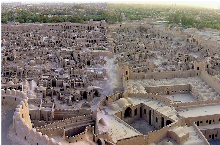
Fig. 87: Bam before 2003 earthquake (Damoun Vahabi-Moghaddam)
