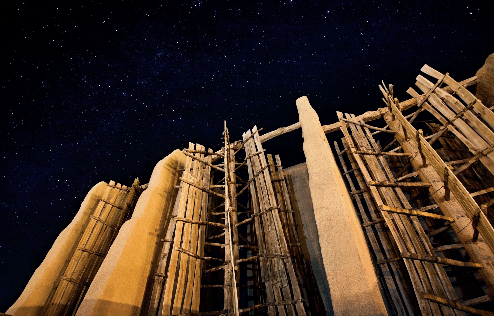
Fig. 135: Application of wind energy in traditional Persian architecture, Nashtifan windmills (Hossein Farahani)
