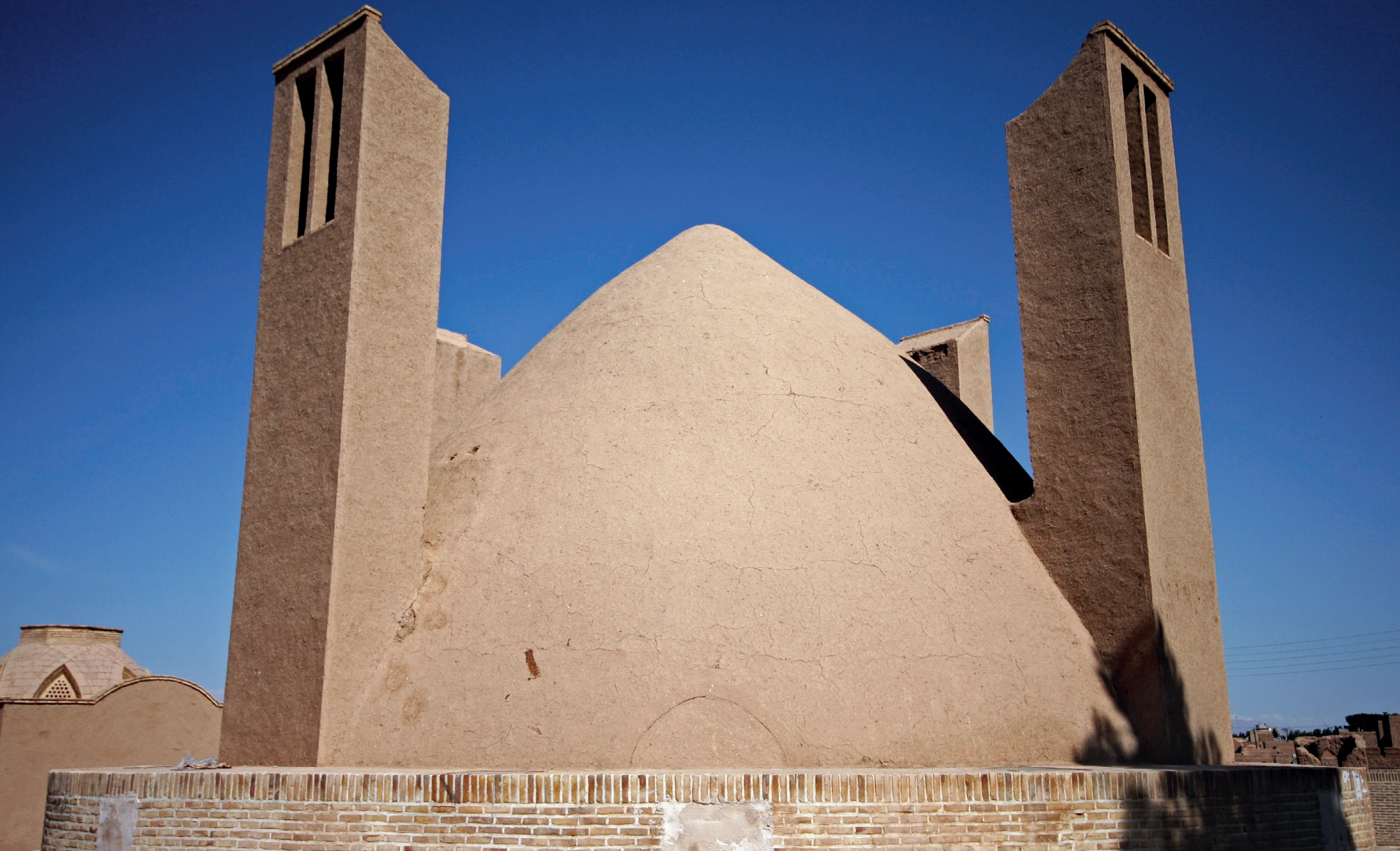
Fig. 134: Application of wind energy in traditional Persian architecture, a water reservoir (Ab-anbar), Meybod (Hossein Farahani)
