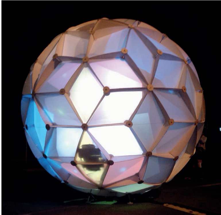
Fig. 89: Spherical structure with fewer elements in comparison to geodesic, diameter = 4.5 m, weight: 180 kg, "Hybrid Globe" interactive installation at Scotiabank Nuit-Blanche Toronto, 2013, Arthur Wrigglesworth, Mohammad Mehdi Ghiyaei, Mojtaba Samimi
