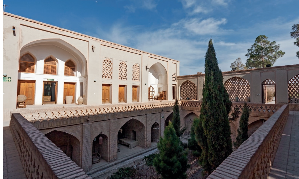
Fig. 131–132: Two different views of local architecture in humid and dry climates in Iran; above: Sobatan village, Talesh, below: Pirnia house, Nain (Hossein Farahani)
