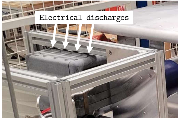
Figure 13-5 LV frame top side electrical discharges
