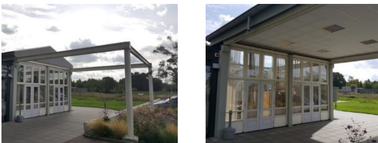
Figure 1-1 Classroom with a retractable roof. The left picture shows the roof covering the classroom. The right picture shows the roof in the retracted position (Photography: Mark P. Mobach).
