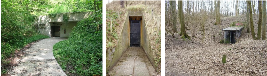
Figure 2. Current eye's nitrate bunkers. 1) Overveen; 2) Heemskerk; 3) Castricum.
