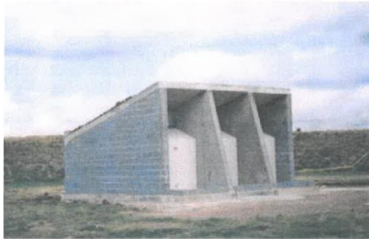
Figure 32. Exterior view of front of facility.
