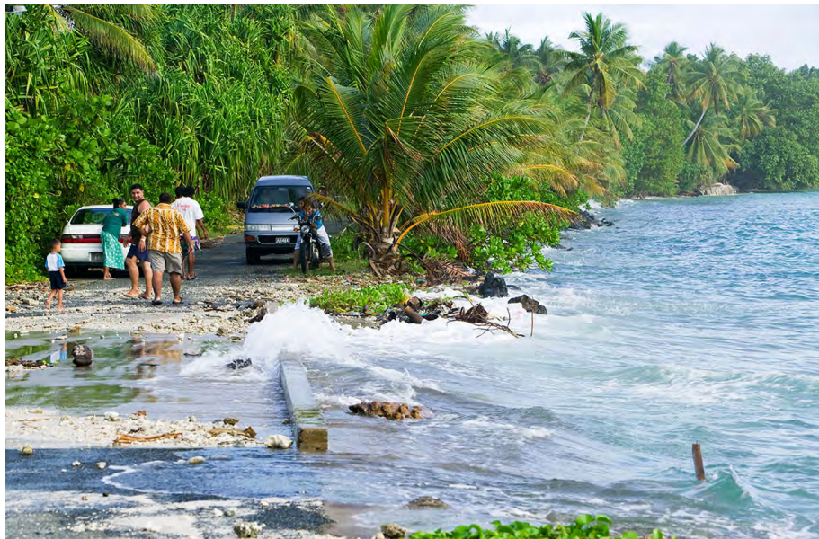
Figure 4. Sea level rise affects infrastructure
