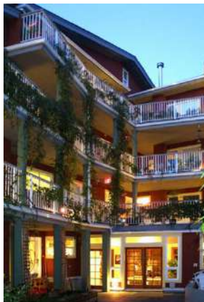
fig. 5 View to courtyard
