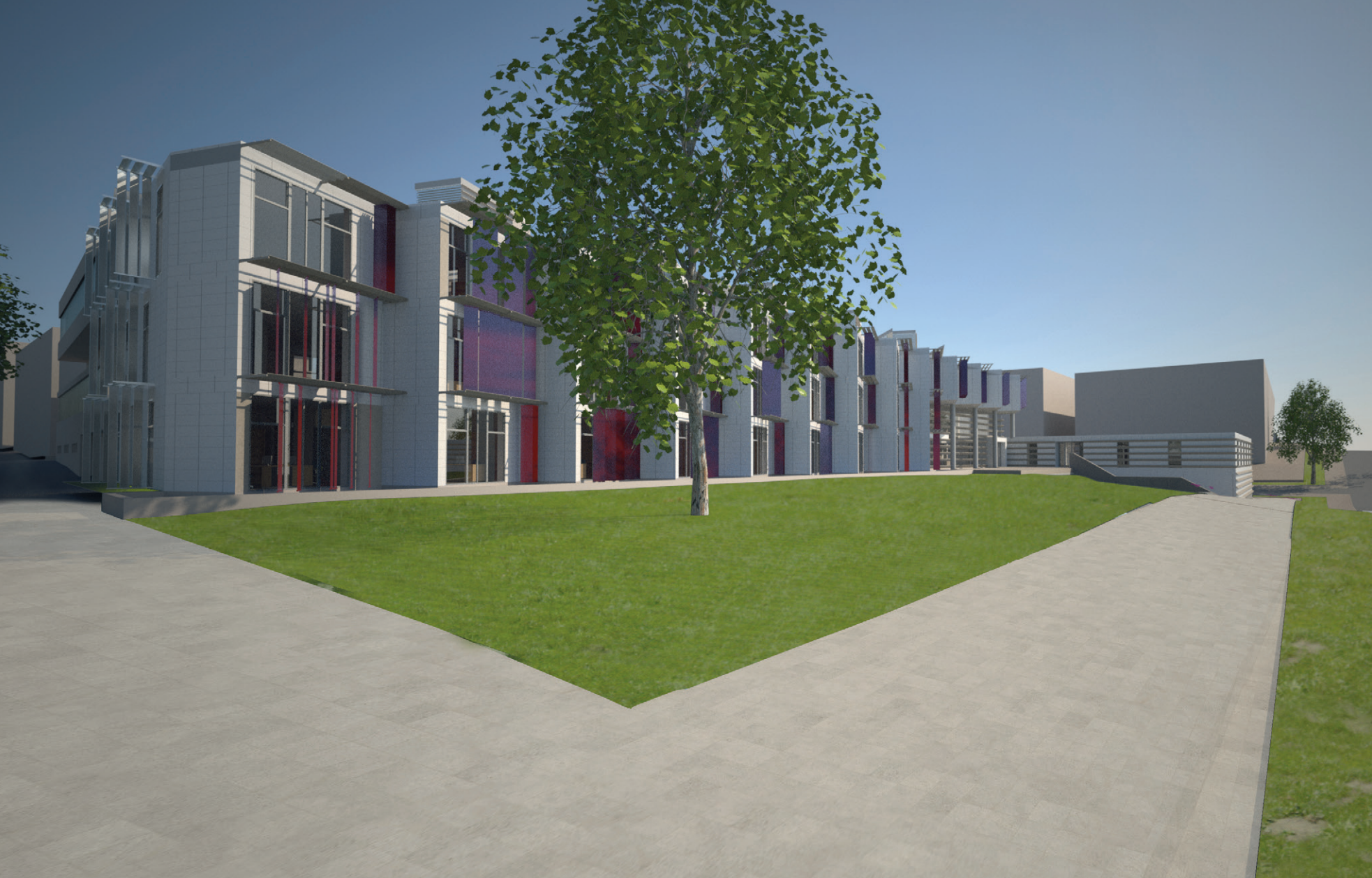
Fig. 115: South-west view of the New Generation Office Building
