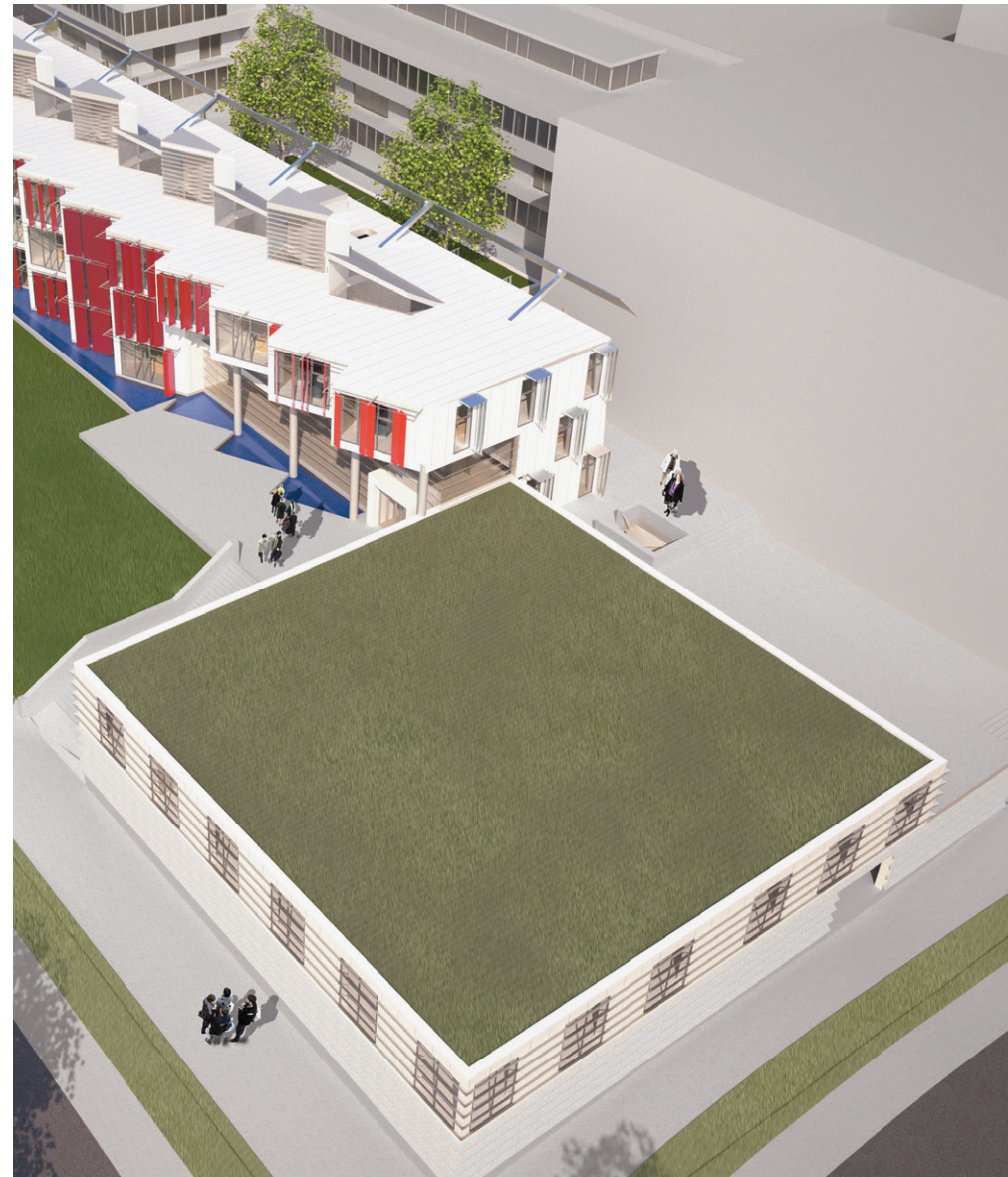
Fig. 78: Green roof on the eastern part of the building
