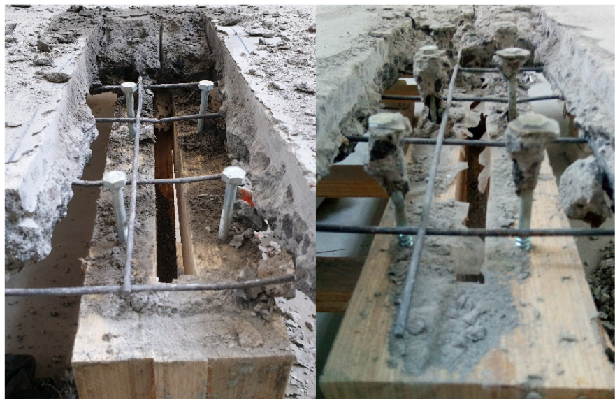
Figure 13. Shear connector after loading test.
