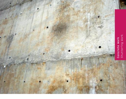
Poor quality concrete surface due to improper shuttering and/or use of too much bond breaker
