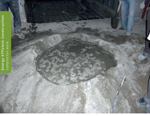
Improper manufacturing of the floor screed, making the correct mix proportion impossible Insufficient mixing Mixing of the floor screed at the job site Uncertain quality and physical properties
