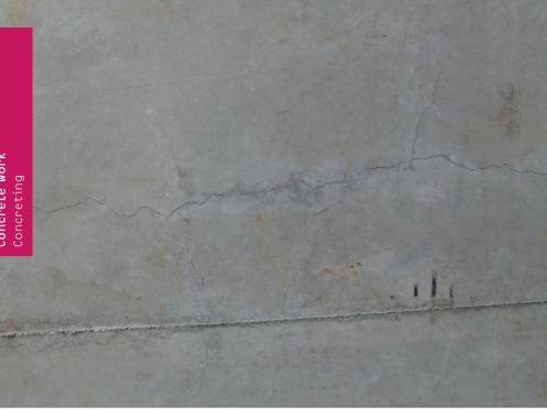
Contraction cracks located in new concrete ceiling Improper concreting, i.e. removal of shuttering too early, too quick dehydration, wrong concrete additives
