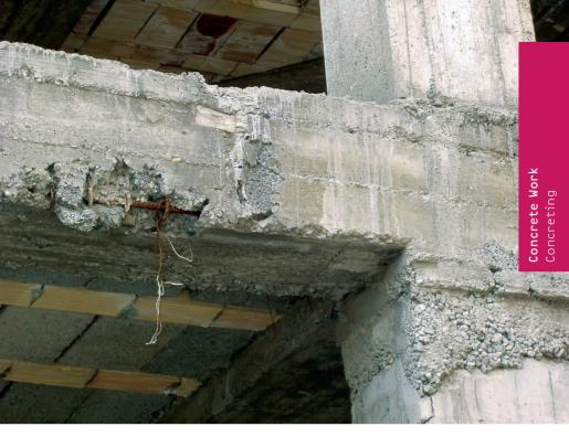
Exposed reinforcements, clearly visable concrete transitions (ceiling—column), incorrect concrete composition, poor compression Poor and imprecise shuttering transitions
