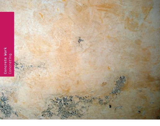
Improper shuttering, inadequate compression (lower edge in the picture) Wrong concrete recipe
