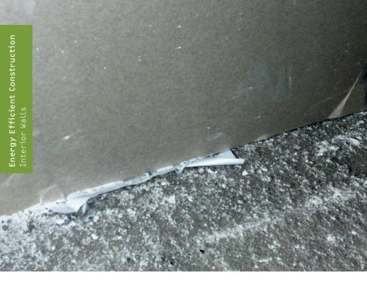
Improper connecting arrangement: gypsum cardboard is placed on the raw ceiling Screw head punctured the gypsum cardboard (screws are screwed in too deep)
