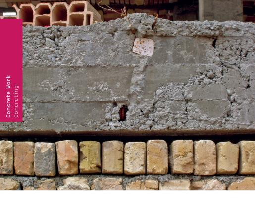
Clearly visible hollows in the concrete, exposed reinforcement, production of concrete with incorrect recipe, poor compression, poor concrete quality, clearly missing supervision of concrete quality
