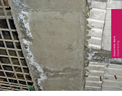
Blooms at the concrete surface, impurities in the components (i.e. chlorides and sulfates), possibly too low temperature while concreting
