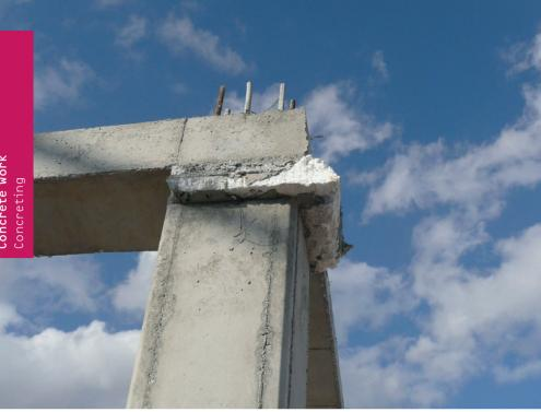
Exposed access bars of the supporting reinforcement (very common in Iran, building will be continued as needed) Steel is left exposed to the elements
