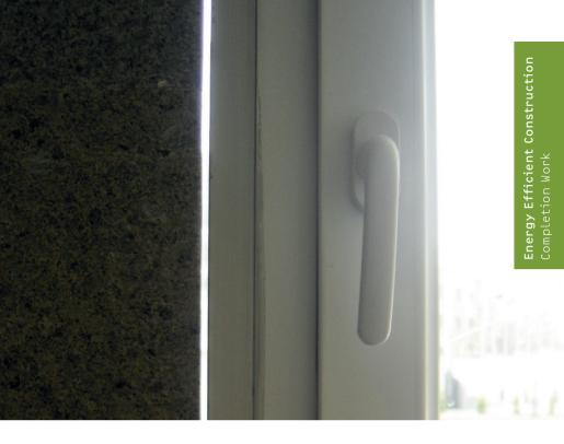
Considerable gap between window frame and masonry No usage of joint material
