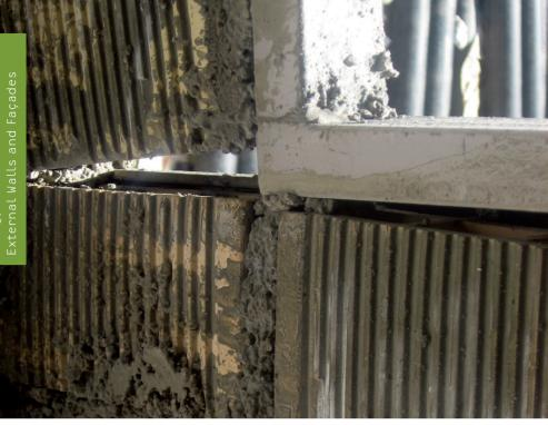
Improper joint structure (partly due to very large joint thickness, missing mortar) No brickwork bond
