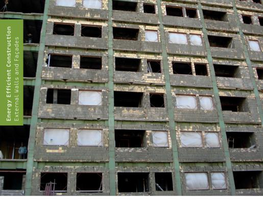
Poor brickwork in terms of quality, heat insulation and construction physics, irregular brickwork bond, grooves are partly too large (straight- and course joints) Thermal bridges due to steel frames used as lintels Partial use of quarry stones for an "optimal utilization" of bricks (saving at the wrong end)
