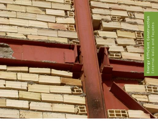
Poor quality brickwork Alignment of the outer wall edge is not uniform Random placement of bricks, some brick openings run straight through the wall Improper connection between brickwork and steel girder Installation of defective material, i. e. bricks No brickwork bond
