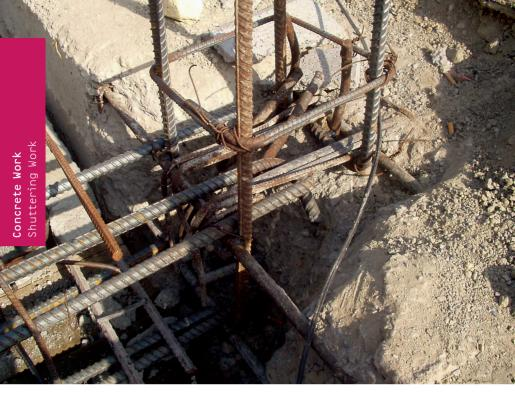
Imprecise reinforcement path with starter bars in an already concrete encased reinforcement Improper transmission of the load from the column to the base via the reinforcement
