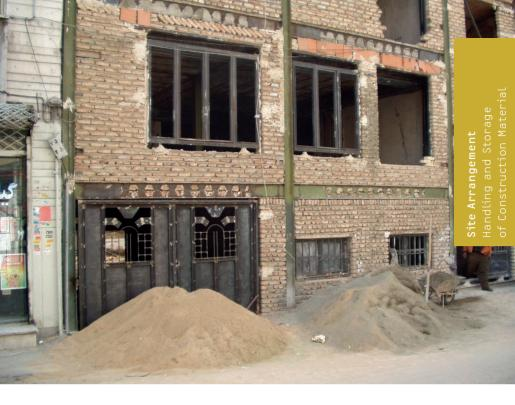
Improper storage of construction material and construction waste Construction material and construction waste become partially mixed
