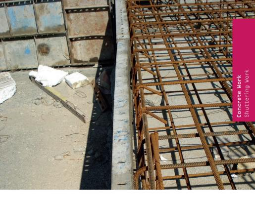
Uneven space between reinforcement and shuttering due to missing spacer Usage of different, uncompatible shuttering systems Missing connections between shuttering elements (unprofessional connection with wire)
