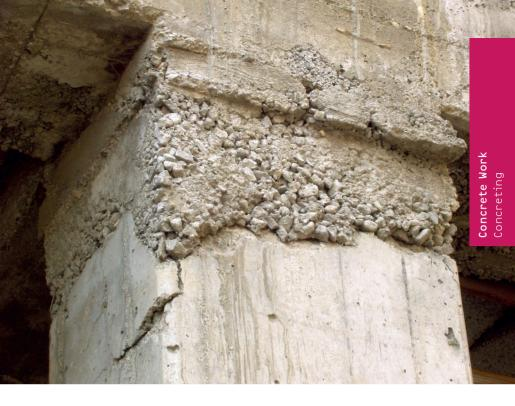
Improper shuttering connection, incorrect consistency, erroneous mixing ratio Improper scaffolding work
