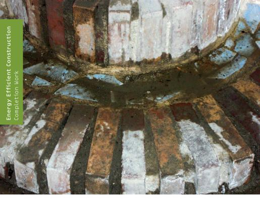
Improper execution of the arch Unevenly laid fraction tiles Uneven joint alignment Sample from the training workshop (bad example)
