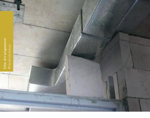
Missing mounting elements for the air conditioning canals Mounting the canals on the wall leads to missing connection between ceiling and wall
