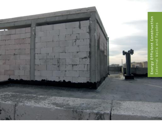
Improper execution of wall connections (no connection between wall and ceiling)
