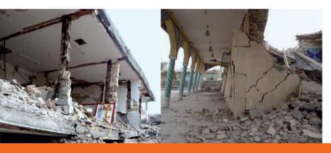
the ceiling, no convenient support for beams and end spans and no tie beams underneath the ceiling. Thus, the damage seen in these ceilings was actually entirely predictable.
