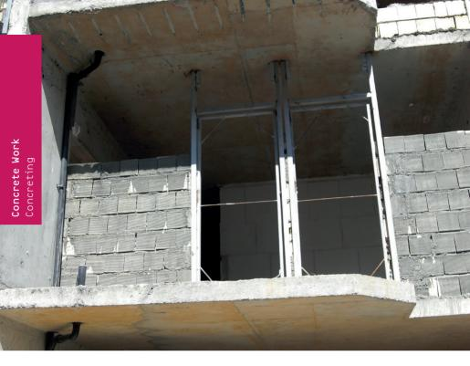
Inadequate concrete compression, consistency of concrete mix too stiff No concrete coverage, position of lower reinforcement visible (bottom of balcony slab), no or incorrect spacers used
