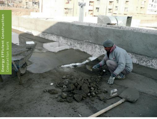
Deconstruction due to improper workmanship (happens often at Iranian construction sites) Execution errors caused by deficient planning and/or supervision of work
