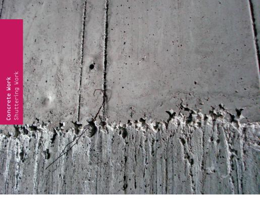
Unsatisfactory execution of shuttering work Incorrect execution of transitions Improper concrete consistency
