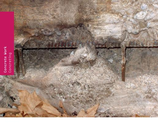
Exposed reinforcement, no concrete coverage Inapropriate or incorrect concrete recipe Poor or missing concrete compression
