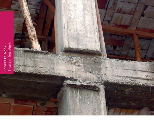
Usage of different shuttering systems Improper shuttering execution Inadequate concrete quality
