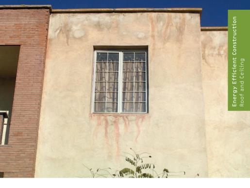
Clearly visible plaster discoloration in the upper part of the masonry, underneath the attic and windows Attic is not covered with weatherproofed material Insufficient covering, missing drip edges, insufficient overhangs No window sills
