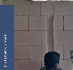
Chiseling channel slots into the new wall in order to install power supply lines/empty conduits Improper execution of AAC masonry
