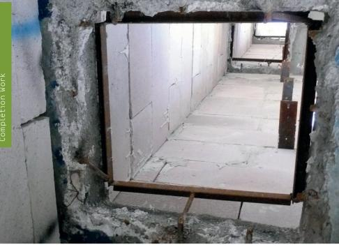
Poor floor breakthrough Steel frame subsequently welded on to the reinforcement of the ceiling Exposed, broken reinforcement
