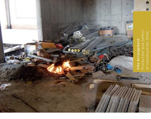
Unorderly and improper storage of construction materials Open fire at the construction site to warm up construction workers
