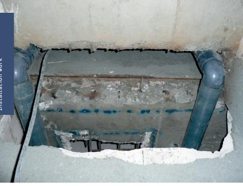
Breaking through the ceiling to lay pipes Unacceptable severing of the ceiling reinforcement Perhaps missing detailed installation planning
