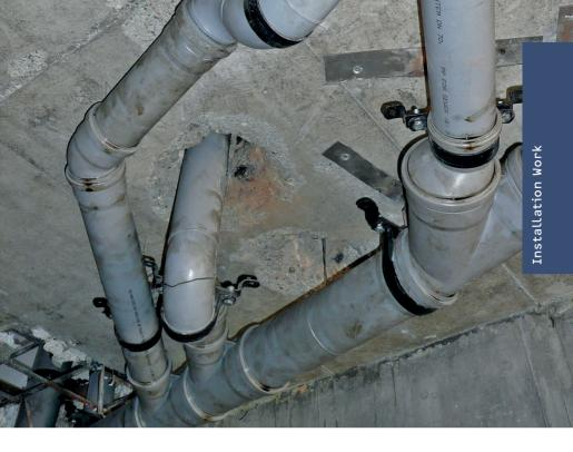
Improper pipe installation—unnecessary bends and bypasses Perhaps missing installation plan
