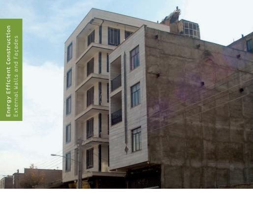
Steel skeleton visible at the pediment Steel girders stick out of the pediment and are exposed to the elements (often visible defect in Iran)
