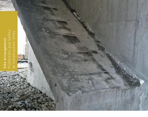
Disregarding occupational safety in shell construction of stairs Missing stair railings as fall protection No safe stair treads (only wire straps)
