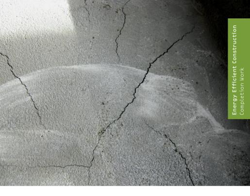
Crack formationin floor screeds surface Incorrect floor screed recipe Improper manufacturing process (i.e. manual mixing on site) Possibly missing reinforcement
