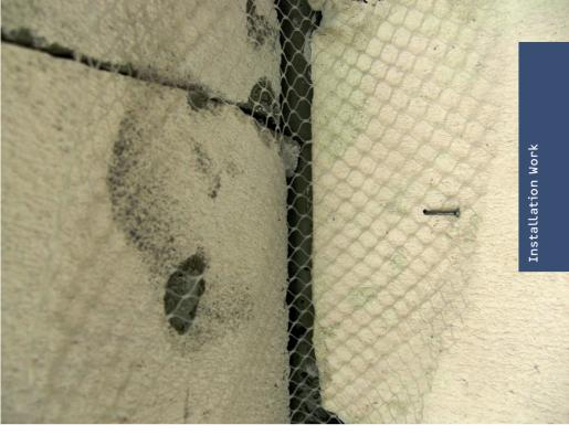
Connection of masonry to concrete column Installed reinforcement fabric for bridging the cracks located in the plaster because the masonry and reinforced concrete have different thermal expansion coefficients Reinforcement fabric mechanically (nailed) attached to masonry
