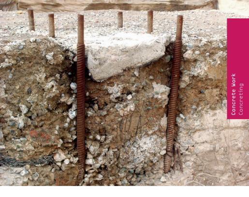
Tie bars are not surrounded by concrete No composite action between reinforcement steel and concrete Incorrect concrete recipe, incorrect granulometric composition of construction aggregates, no concrete compression
