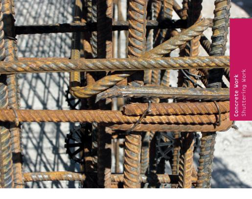
Improper installation of the reinforcement, much too tight (maybe missing information about minimum distances in planning documents) Missing spacer, the concrete can only partially surround the reinforcement
