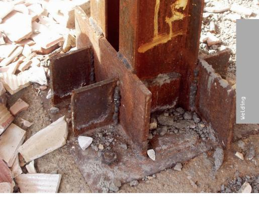
Improper execution of a bracket weld: poor welding seams, poor connections
