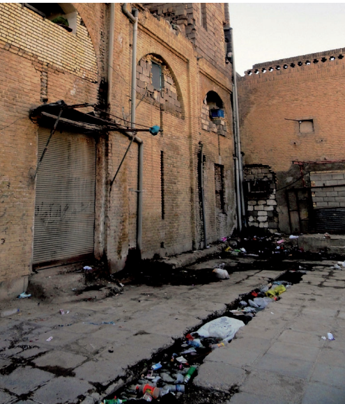
Fig. 32: The lack of urban service: waste is not regularly collected (Author)
