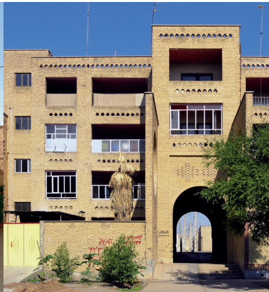
Fig. 37: Balconies walled or added to interior (Author)
