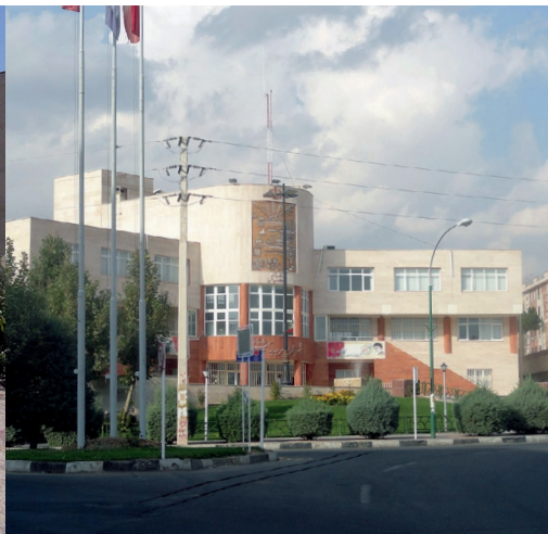
Fig. 50: View to the Municipality building at the central square (Author)
