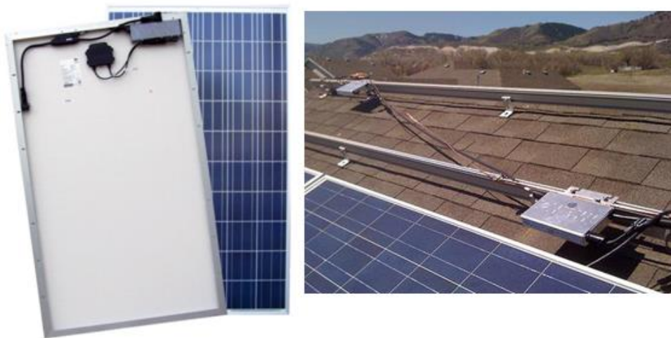
Figure 4.5 Module-integrated (left) and externally mounted micro-inverter (right).
