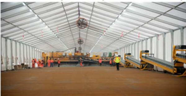
Figure 12. Strengthening by HSC, Kreekrak Bridge
