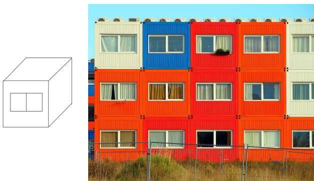
Figure 2.2: Model of a house formed of prefabricated pieces on the left-hand side, and houses made of prefabricated pieces in the real world on the right-hand side.
