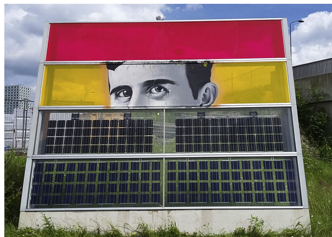
Fig. 10. Photograph after partial removal of street art design on the surface of the LSC panel.
