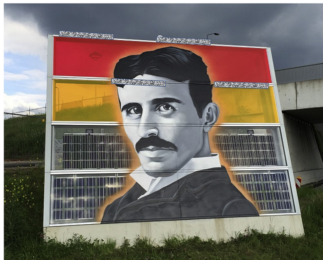
Fig. 7. Photograph showing street art design on the surface of the LSC panel: position of solar strips indicated in the figure by textured bars (LSC artwork courtesy of Gart Smits, photo courtesy Stijn Verkuilen).
