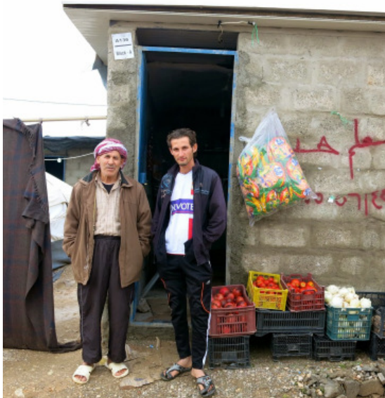
T5. Cement block shelter - Morrow, D. (2014)
