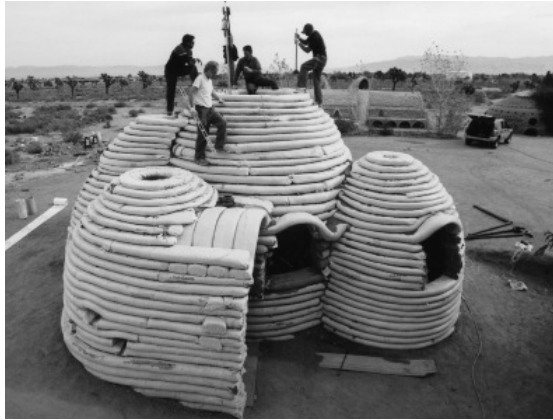
P6. Home built with earth-filled sandbags
