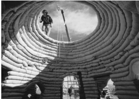
P7. Building process
