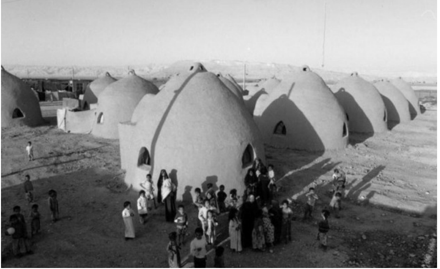
P9. Sandbag shelters with plaster finishing in Baninajar refugee camp, Iran. Constructed in 1995 and demolished in 2012
