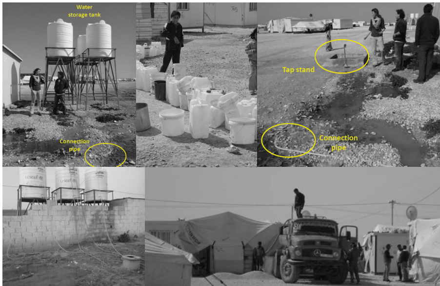
Z4. Distribution of water at private connections. All distribution points in Za'atari can be found in the letter O rganisation).
