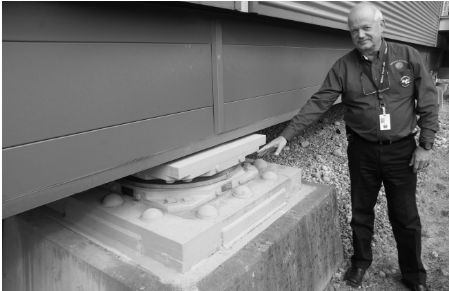
D2. Chris Utzinger points to the earthquake-resistant piles - Forewarned.info, 2016
