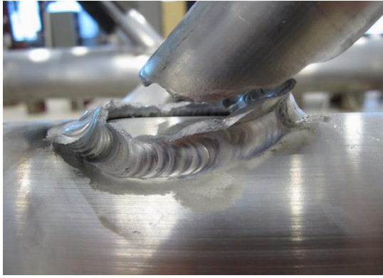
Fig. 10: Failure in heat affected zone of diagonal 1
