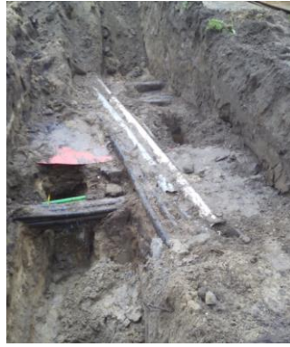
Figure 6. Underground utilities together with the red cover in the test trench
