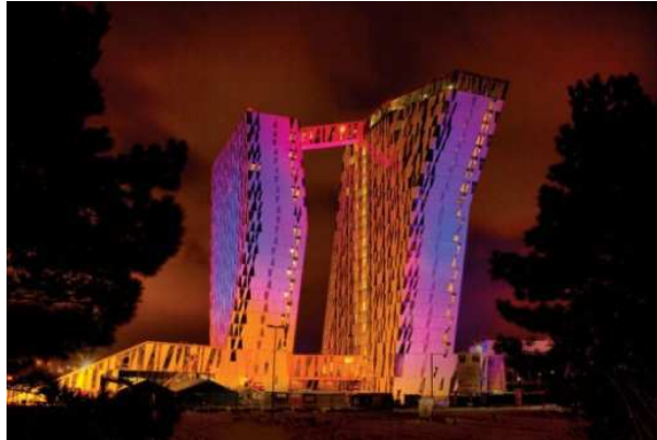
FIGURE 5.19 BELLA SKY COMWELL HOTEL. COPENHAGEN, DENMARK
