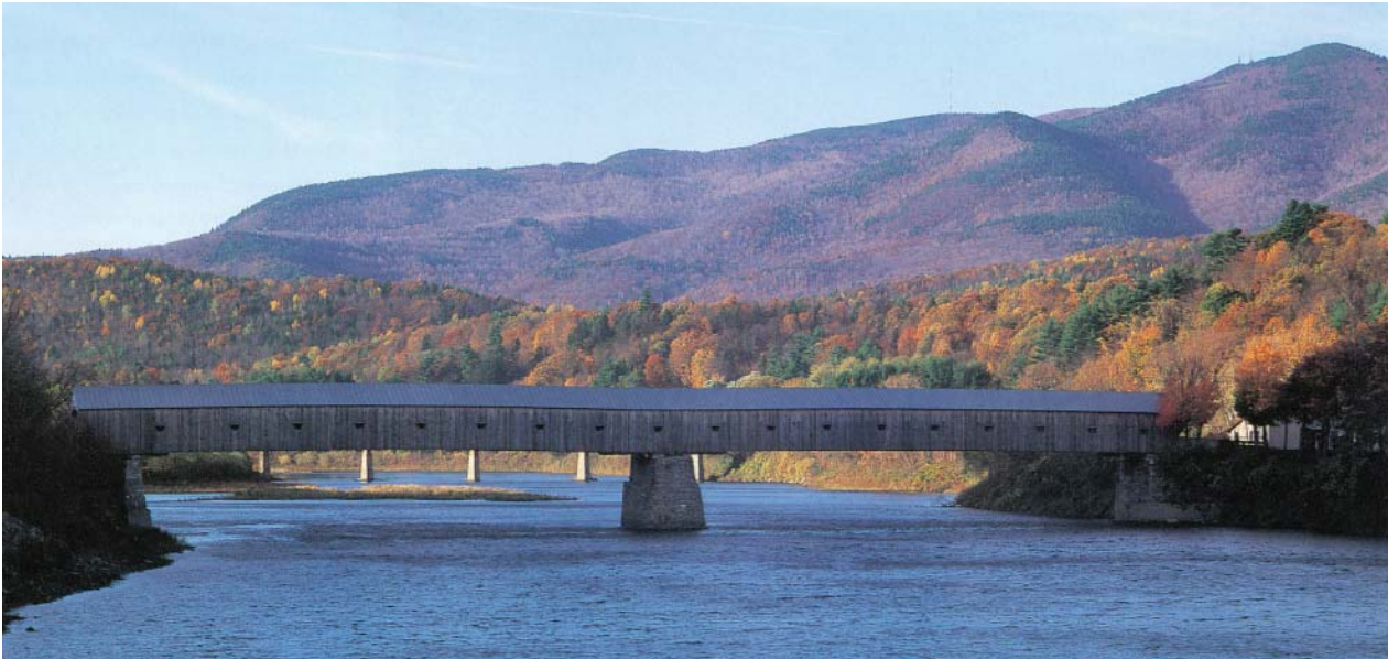
Cornish/Windsor bridge, Sullivan county, New Hampshire, USA
