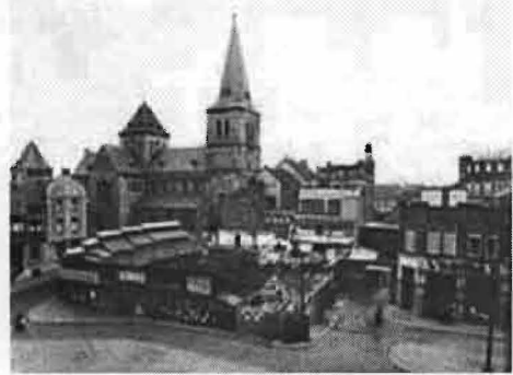
Figure 1.2: The Glasspalace under construction
