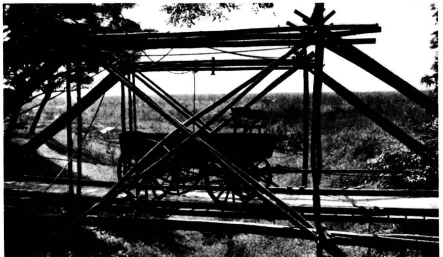
The Bridge under a 3,500-pound Load
