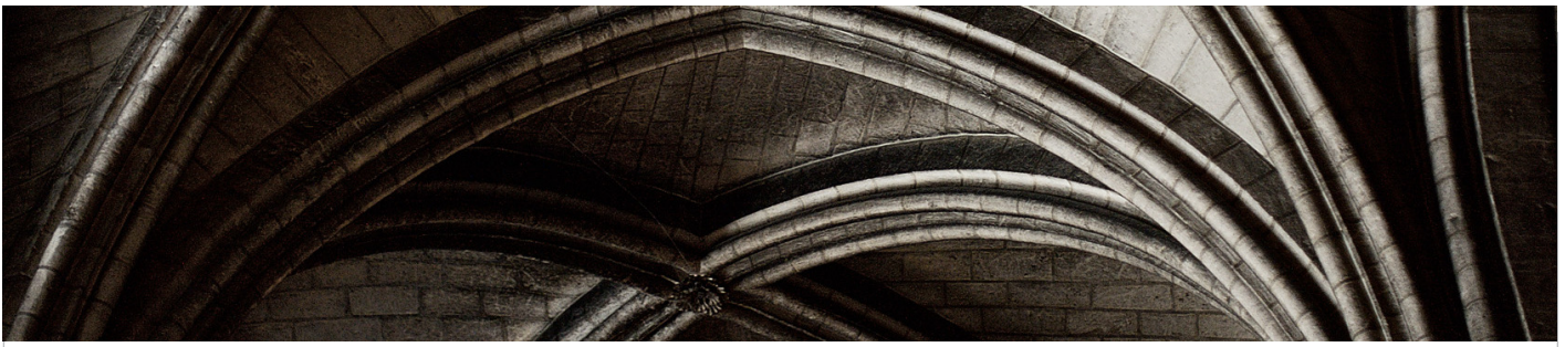
img 1 | Cross-ribbed vault
