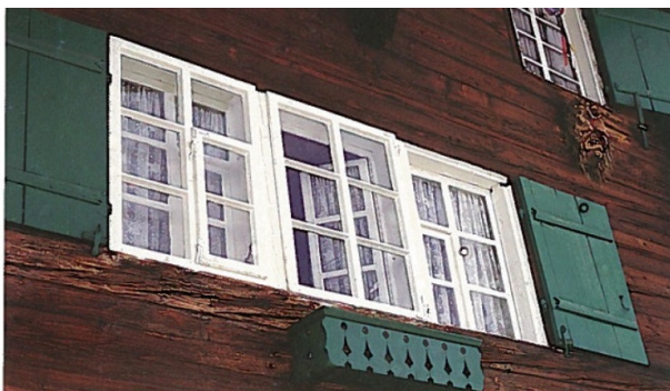
Figure 2.1. Façade of an old farmhouse with box windows
