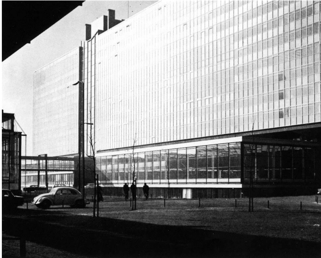
Figure 4.7. Photo of the Main Building, date unknown (source:OD205 architectuur)
