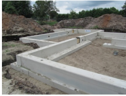
Figure 2. Precast strip footing (1)
