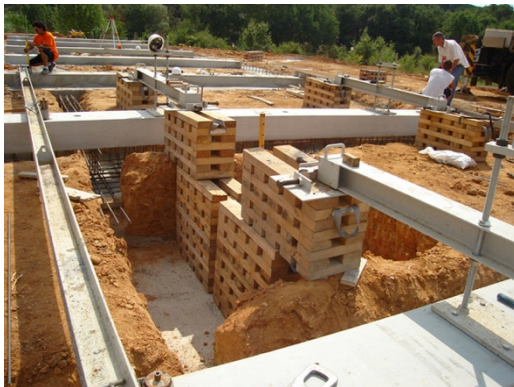
Figure 14. Lower beam parts were built in situ. The section was variable. Figure 15. Lower beam parts were reinforced with steel.
