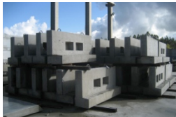
Figure 3. Precast strip footings (2)
