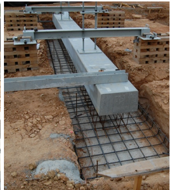
Figure 14. Lower beam parts were built in situ. The section was variable. Figure 15. Lower beam parts were reinforced with steel.
