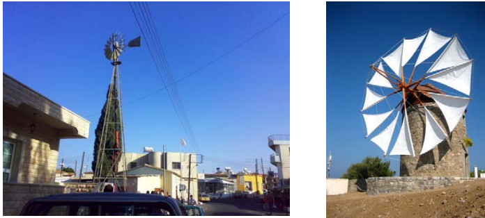
Fig. 2: Old wind energy systems used in Greece and Cyprus for water pumping and grain grinding
