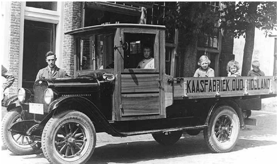
Figure 3.2 Truck body made by wagon maker Jan van der Roest, IJsselstein, 1927.
