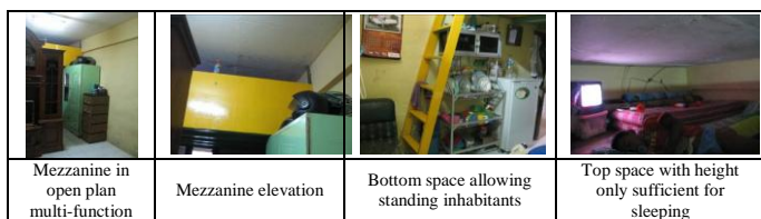
Figure 9. Illustration of mezzanine construction
