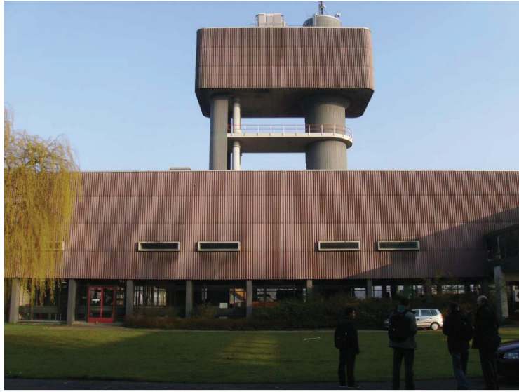
Figure 3: The water tank with a constant 25 m head at Deltares, Delft, The Netherlands. It has been brought down in 2011.
