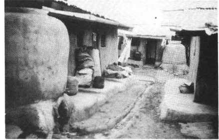
fig. 3.2 Squatter-unit upgrading project, Kinyago village, Nairobi
