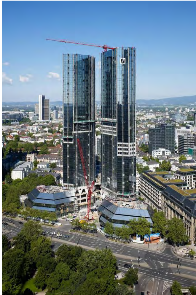
Figure 1.3. Deutsche Bank headquarters in Frankfurt am Main during refurbishment (DB Greentowers 2009)
