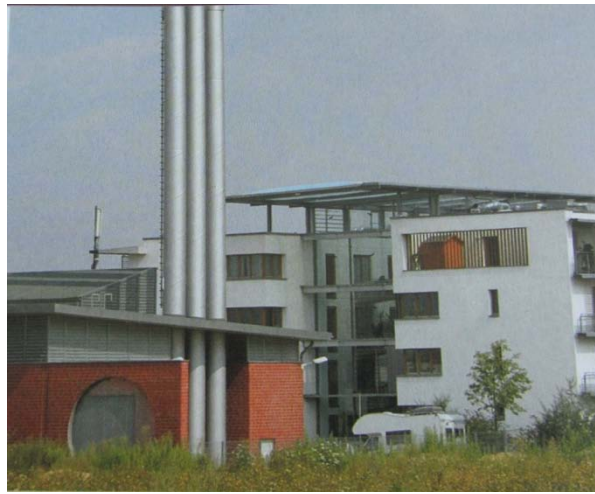
Figure A-1-10: CHP plant in Kronsberg, Hannover
